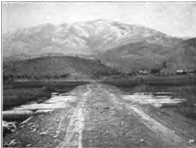
OLD TIMBER CULVERT, STATE ROAD NEAR MARYSVALE, PIUTE COUNTY.
